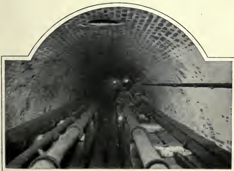
A LONG STREET IN THE SUBWAYS (CHARTERHOUSE STREET).
