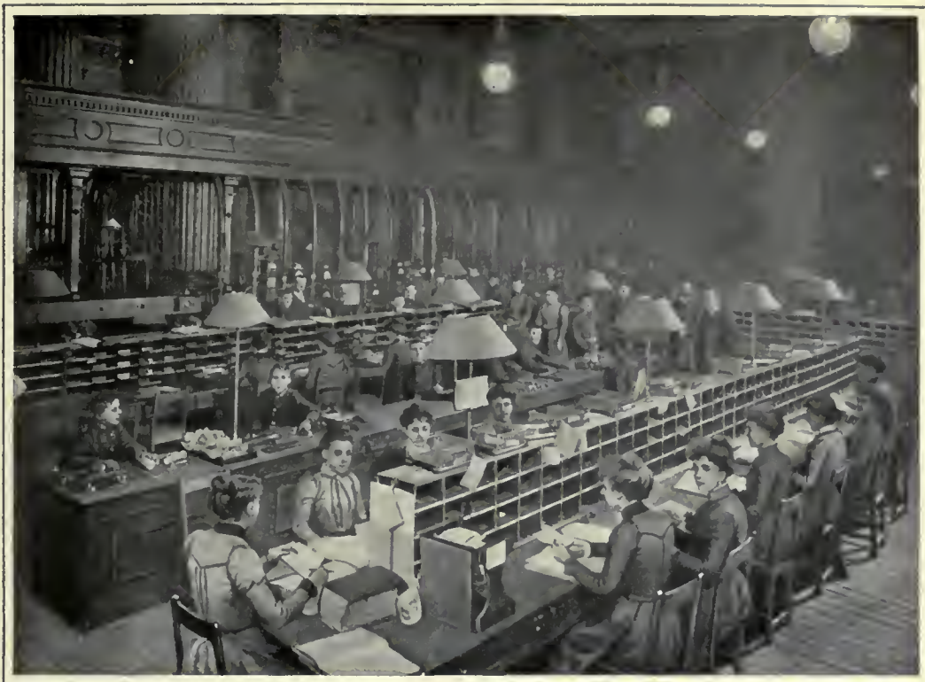
THE PNEUMATIC TUBE ROOM (ST. MARTIN'S-LE-GRAND).
