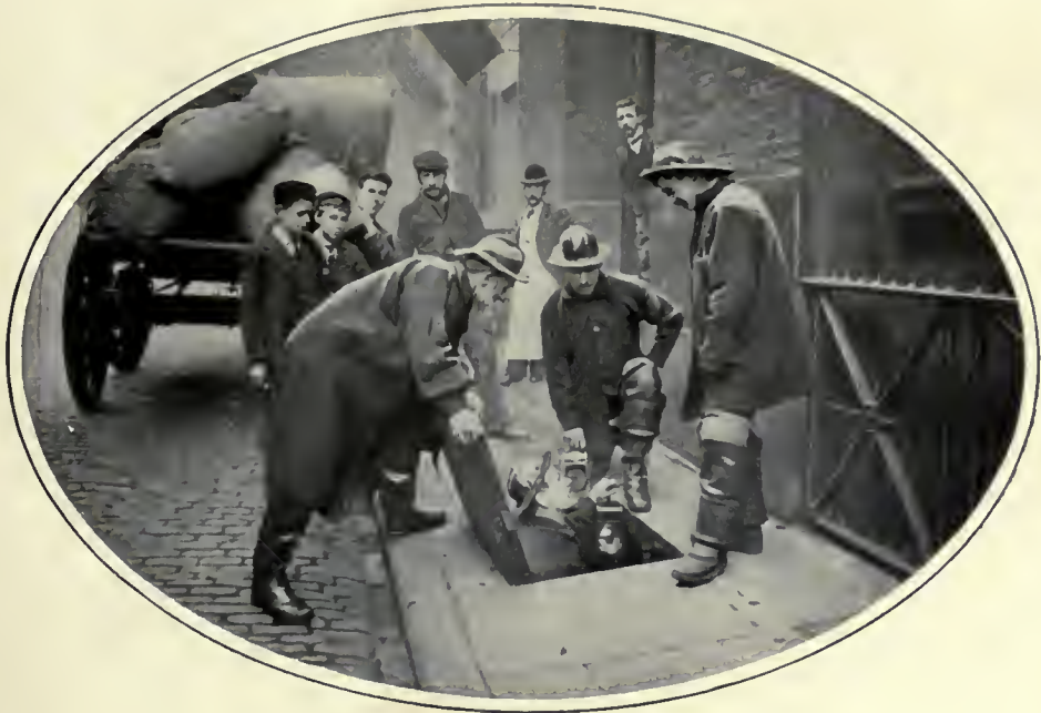
SEWERMEN GOING BELOW.
