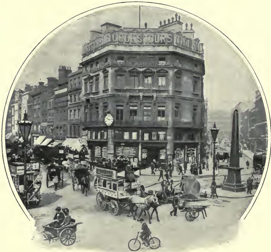
FLEET STREET CORNER (LUDGATE CIRCUS).
