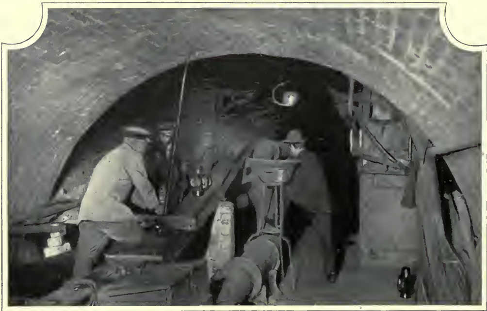
REPAIRERS IN THE SUBWAYS (NEAR HOLBORN CIRCUS).
