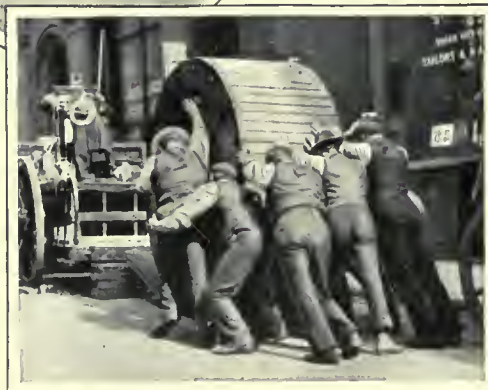
I. WIRE REPAIRERS AT WORK. II. A REEL OF WIRE.
