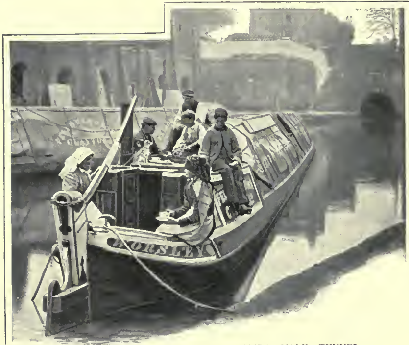
OUTSIDE MAIDA VALE TUNNEL.
